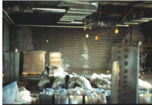
Expansion joint leak
